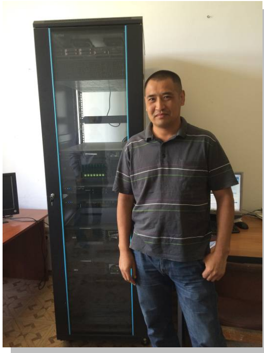
DWRLI IT Staff in the Server Room
